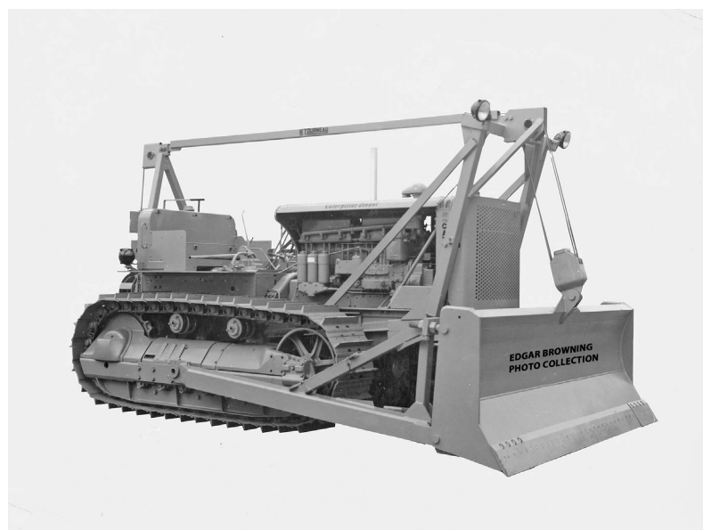
Caterpillar D8 påmonteret en LeTourneau Dozer and Cable layout-skraber. (Foto: Edgar Browning)
