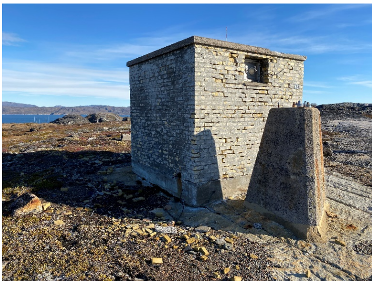
Fig. 15. B-451, the former NDB antenna adapter housing along with a precast cement pylon that served as a mast anchor (foundation element F008), facing southeast. Photo: Harmsen 2020.
