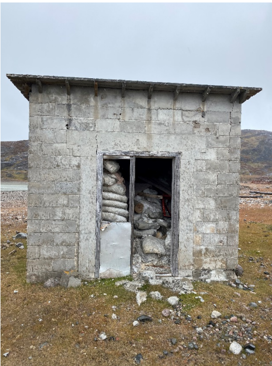
Fig. 104. Building B004, showing concrete mix sacks that have solidified and now become a permanent part of the structure. Photo: Harmsen 2020.
