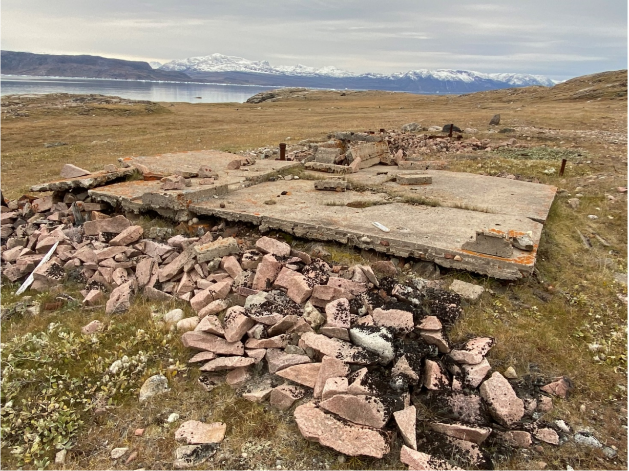
Fig. 88. F002 at Artillery Point. The cement platform is in extremely poor condition, with visible breakage and cracking due to exposure to the wind, rain and ice over the last 70+ years. Photo: Harmsen 2020, facing south.
