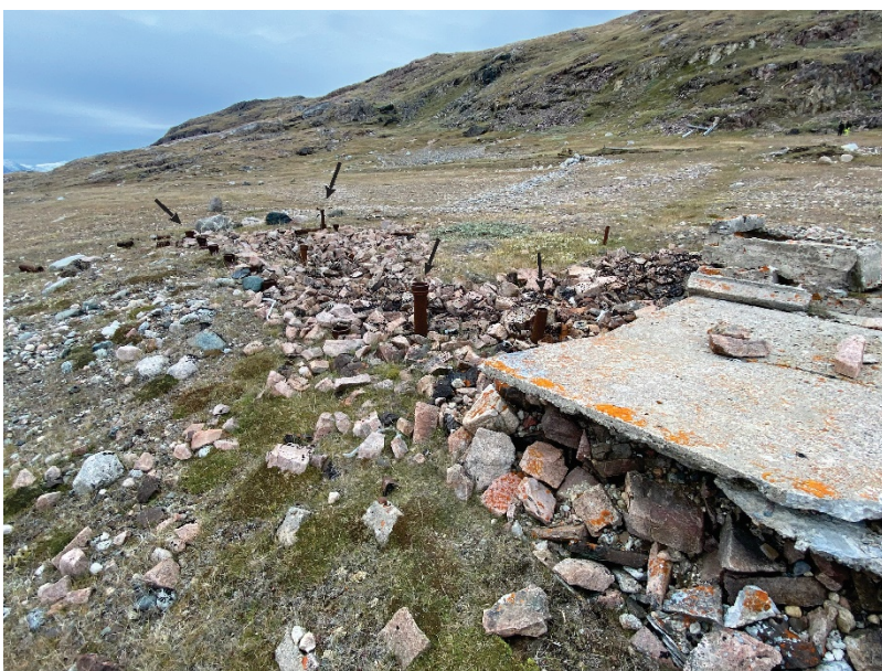
Fig. 87. Several infrastructure elements such as exposed plumbing and pipe fixtures are found in connection with F002. Arrows point to exposed pipes. Photo: Harmsen 2020, facing southwest.
