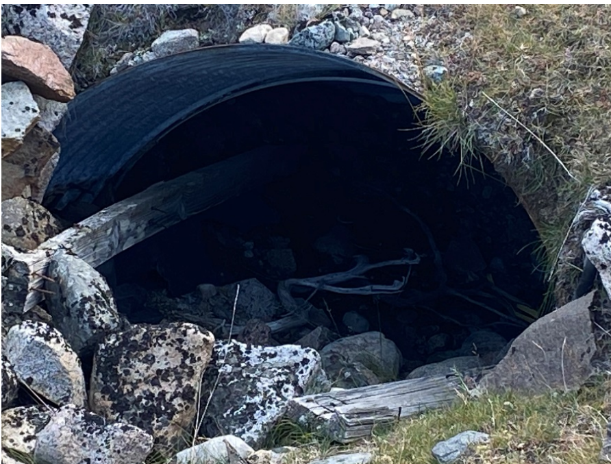
Fig. 77. Entrance to D007. The roof of the entrance was supported with a concave corrugated steel fitting. Several pieces of scrap wood and debris were present in the entrance. Photo: Harmsen 2020.
