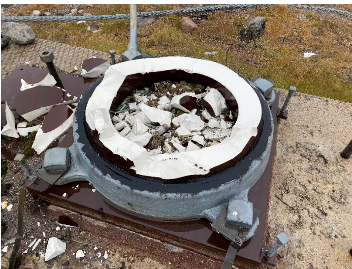
Fig. 112. Ceramic insulator base of the steel antenna mast. Photo: Harmsen 2020.
