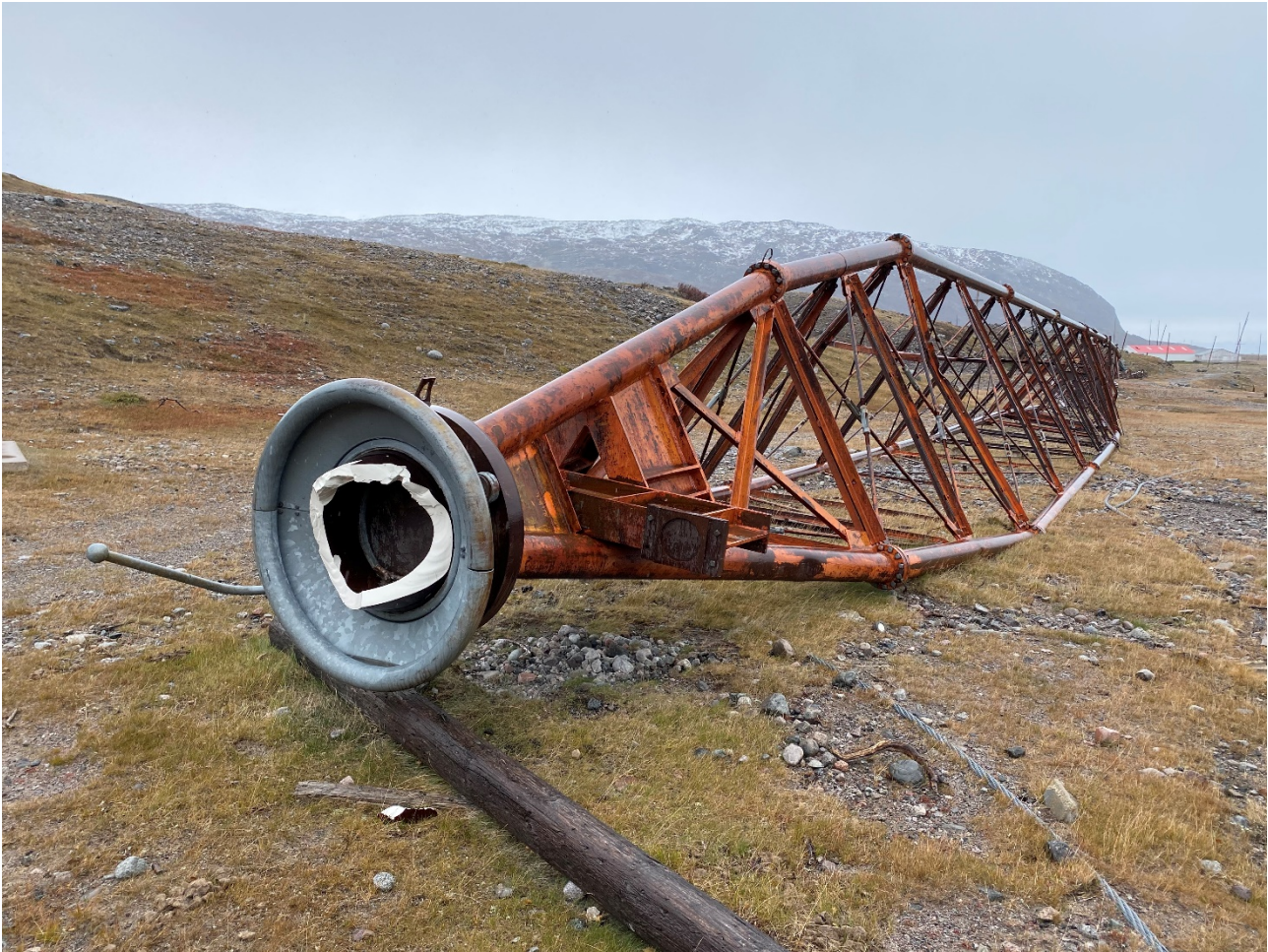
Fig. 111. The steel monopole antenna mast at Camp Corbett originally stood at a height of 185 m above the ground. The mast have been left in place along with remnants of its various components. Photo: Harmsen 2020.
