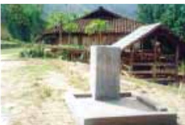
Vietnam : a pilot project in Thai Nguyen, constructed a system to ensure a safe water supply Photo : Committee for Ethnic Minorities in Mountainous Areas (CEMMA)
